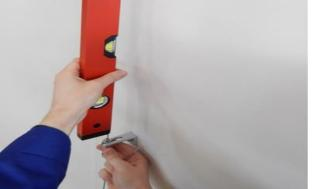
6. Install façade tightener to the bracket.
