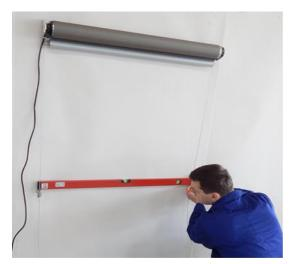
11. With a spirit level mark the installation place of the second cable guide bracket. Other actions make analogically to the first bracket and guide.
