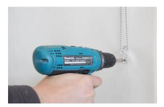
Tightened chain should be installed to the wall with the use of safety bracket – at height 150 cm minimum above the floor. If necessary adjust the chain length.
