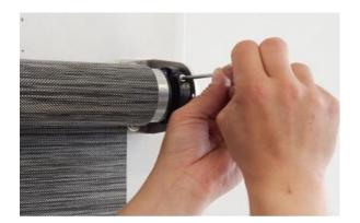
In niche installation connect first the wall-ceiling bracket to the drive, the with already fixed bracket install the blind in the niche.
