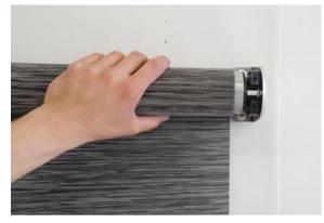
4. Mark places for openings and install to the wallceiling second bracket.
